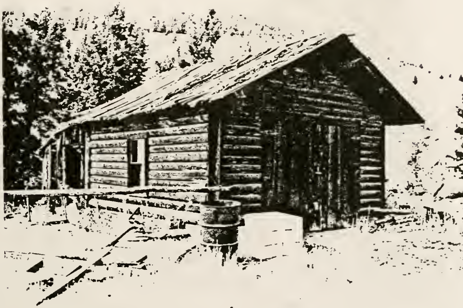
Figure 211. Structure #92, northwest view.
